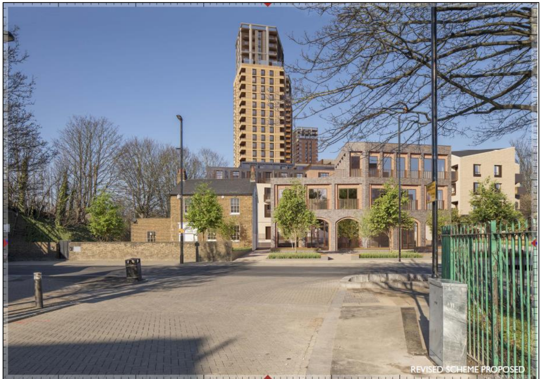
Western pavement of Love Lane (outside WHL Station) looking north (View 24)
