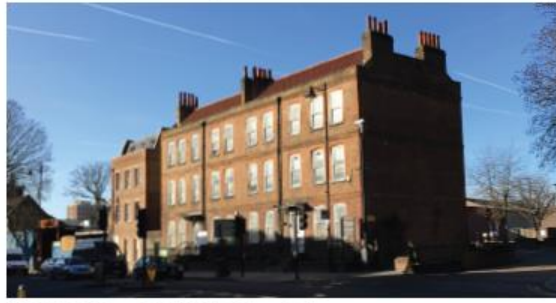
FIGURE 42. - 867-869 High Road (C)
