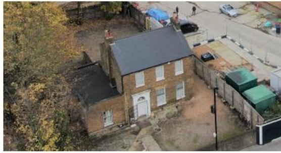
FIGURE 40. - Station Master's House (A)
